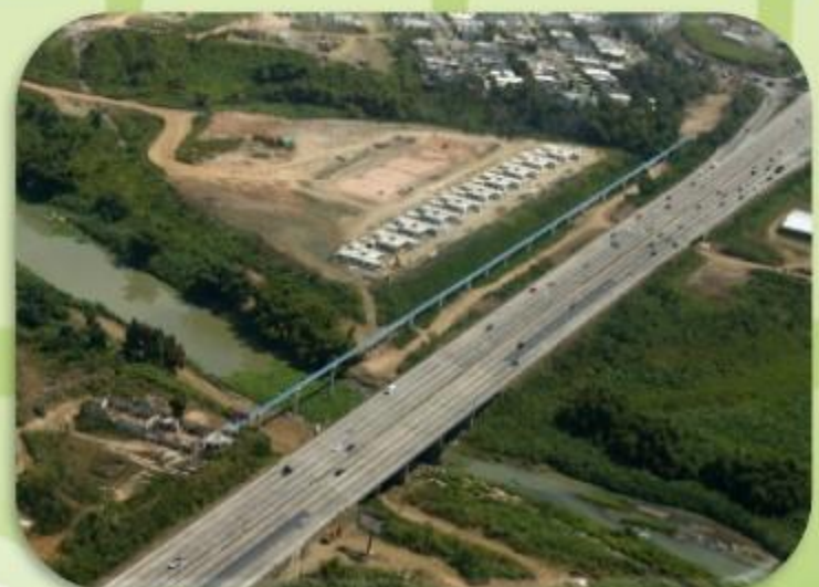
30" PIP M.G. WATER TANK, GURABO, P.R.
