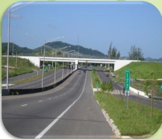
BRIDGE OVER PR-2 AS PART OF THE INTERCHANGE WITH PR-3362
