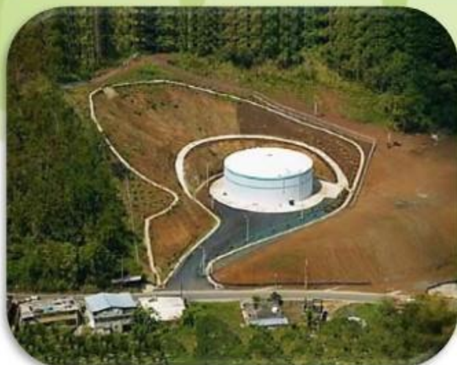
2 M.G. WATER TANK, GURABO, P.R.
