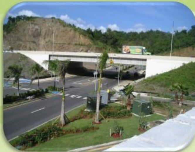
BRIDGE OVER PR-2 AS PART OF THE INTERCHANGE WITH PR-122
