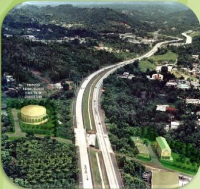
PIEDRAS BLANCA TANK & PUMP STATION, GUAYNABO, P.R.
