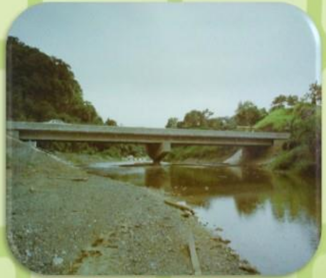
BRIDGE OVER ROSARIO RIVER SAN GERMAN
